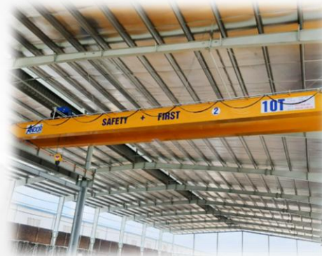
INSIDE CRANE 10TONS
